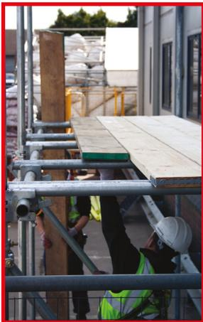
Altrad Generation Readylok Transoms are made to predetermined sizes, fully plated, with preset vertical and horizontal couplers to enable standards and ledgers to be perfectly positioned. This saves a considerable time in measuring and setting out. The result is a fast and fool proof system with its own, high, built in safety factor.
