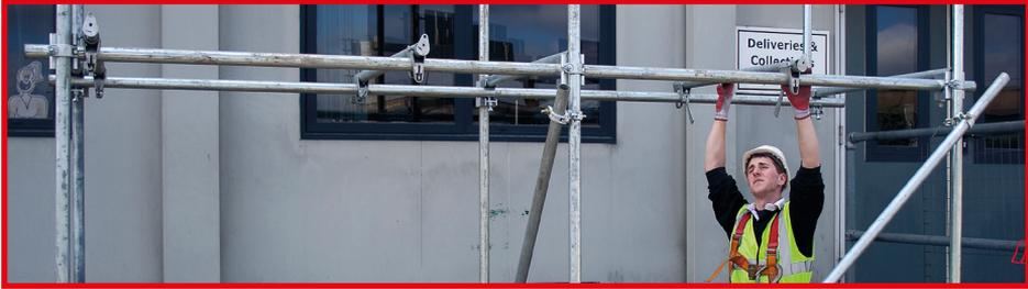
Altrad Generation Readylok Transom units will, at low cost immediately convert your stock of tube and fittings into an easily and speedily erected system scaffold, whilst maintaining TG20 compliant. The use of these pre-coupled units dramatically eliminates the need for loose fittings. In use they will considerably speed erection times reducing labour cost and site losses.
