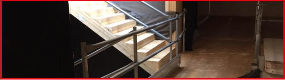
Protecting Staircases can be a challenging task as dimensions can vary. All of our Staircase solutions are supplied with unique Telescopic handrails meaning there is no need to cut down traditional tubes to the required sizes.
