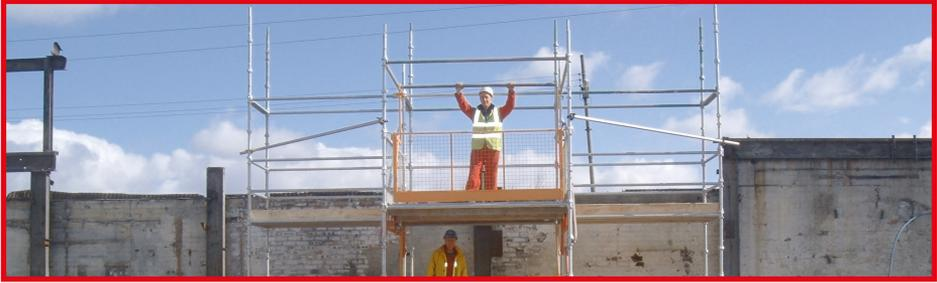
Genlok can be used to create Loading Towers for the purpose of distribution of pallets of materials to the working level by site forklift or loader.
