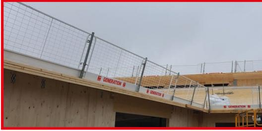
Altrad Generation provides a full range of components for hire for the timber frame edge protection. Like with our steel frame edge protection, you can install our components for Timber Frames on the ground making installation safer and more efficient. We are also able to supply you with top fix solutions and side fix solutions and handrails or mesh barriers can be used.
