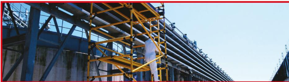
GRP Zone 1 Tower is specifically designed to be used where the use of Aluminium Towers are not appropriate. Providing a safe, non conductive, clean and efficient full protection tower system.
