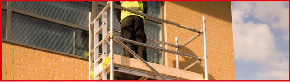
The BoSS Aluminium Tower System is designed to meet users requirements and can be assembled in many different ways to provide safe working platforms for construction industry or inspection/maintenance purposes.
