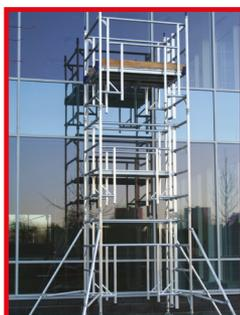
Hierarchical requirements place collective protection over mitigation options. As an advance guardrail system the BetaGuard® provides best practice collective protection, but without the manual handling problems currently associated with industry practice.
