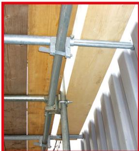
A unique solution for the creation of boarded platforms within traditional tube and fitting scaffolds. Altrad Generation Extendable Intermediate Transoms combines three loose components into one easy to assemble item that is suitable for use with traditional tube and fittings, and with Readylok transoms.
