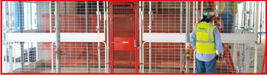
The solution utilises light but extremely robust and user friendly components and features a secure key activated locking gate. Standard EP components such as the innovative Post and Panel are utilised when completely securing the protected areas and with no need for any penetration of the working surface, multiple lift / elevator shafts are protected in just minutes.
