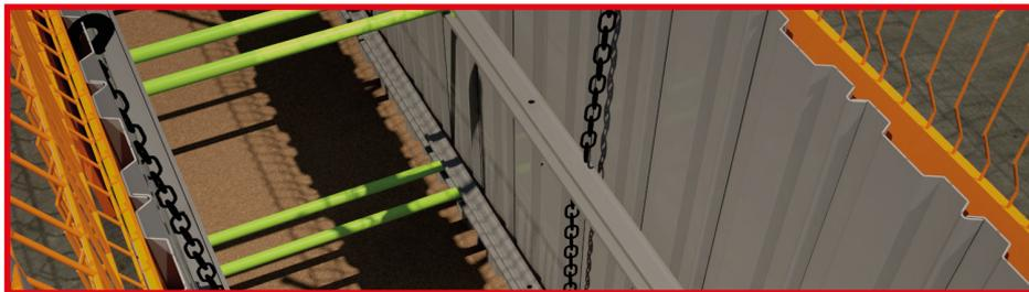
Alloy Waler Rails are used as an alternative to Trench Boxes where cross services are an issue. They are mainly used in city center and highway excavations where ground movement must be kept to a minimum. They offer a two-sided hydraulic support system used in conjunction with Altrad Generation Trench Sheets to allow a clear working area for the inspection/laying of utilities.
