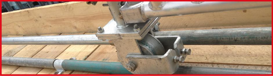
The purpose of the Trax bracket is to provide a cost effective, quick and efficient method for rolling out beam assemblies, gantries or temporary roofs.
