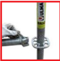
1. Hook in the horizontal ledger
