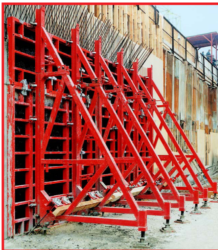
SB-B and SB-C brace frame units with PERI TRIO panel formwork, concreting height 3.50m.
