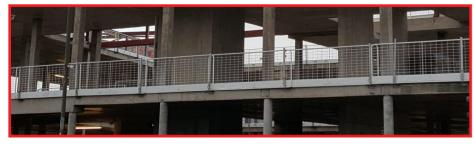
Altrad Generation provides edge protection solutions for concrete frames including systems that don't require any penetrating into the concrete at all. The Rapid Post is a telescopic post that offers single, extended and full containment edge protection using very few components which vastly reduces the installation process.
