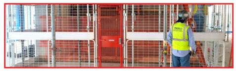
The solution utilises light but extremely robust and user friendly components and features a secure key activated locking gate. Standard EP components such as the innovative Post and Panel are utilised when completely securing the protected areas and with no need for any penetration of the working surface, multiple lift / elevator shafts are protected in just minutes.
