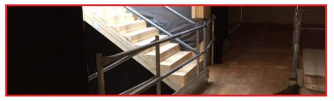
Protecting Staircases can be a challenging task as dimensions can vary. All of our Staircase solutions are supplied with unique Telescopic handrails meaning there is no need to cut down traditional tubes to the required sizes.
