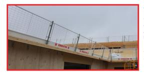
Altrad Generation provides a full range of components for hire for the timber frame edge protection. Like with our steel frame edge protection, you can install our components for Timber Frames on the ground making installation safer and more efficient. We are also able to supply you with top fix solutions and side fix solutions and handrails or mesh barriers can be used.
